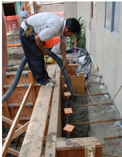
*Pouring the elevator pit walls and footings*
